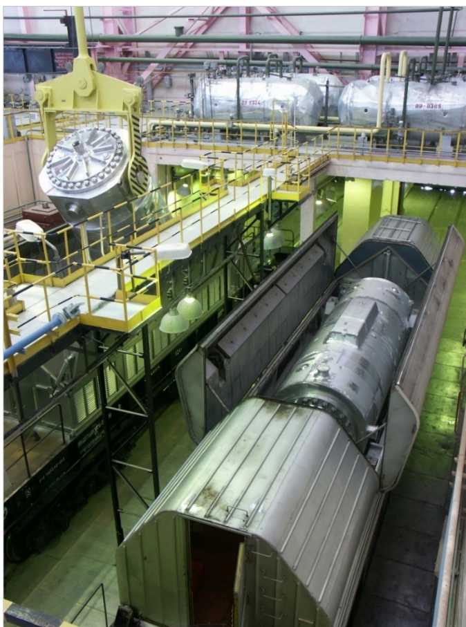
Figure B.2.3 – SNF unloading compartment in the wet storage facility at the MCC site
