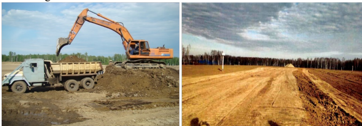
Figure B.4.3 – Backfilling operations at the B-1 storage reservoir (SCC)
